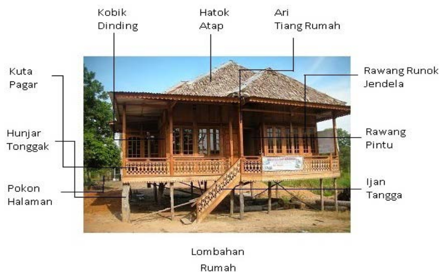
Figure 3.2. Parts of a Stilt House
